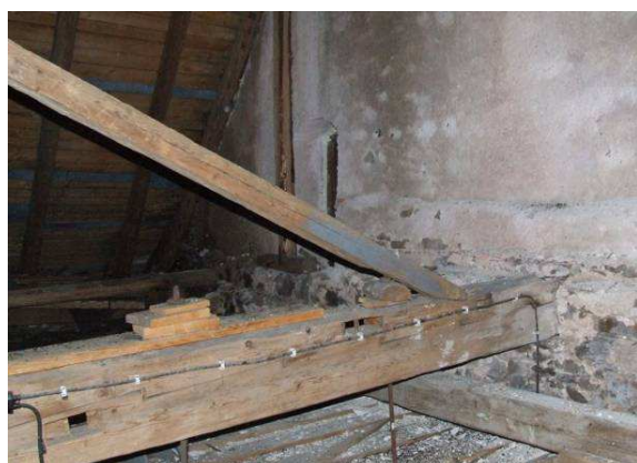
Fig. 7 Left girder anchor beam to the tower walls, right the girder placed on the wall with a visible deflection and tilt to one side.
